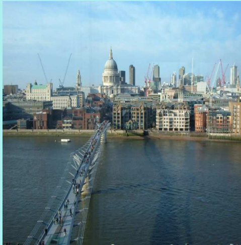
Figure 3. London's Millenium Suspension Footbridge over the Thames.
