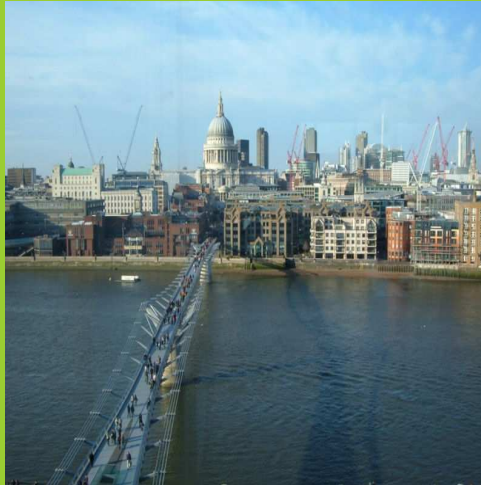
Figure 3. London's Millenium Suspension Footbridge over the Thames.
