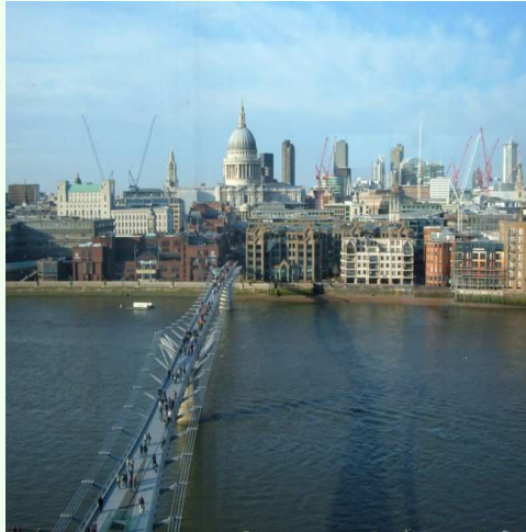
Figure 3. London's Millenium Suspension Footbridge over the Thames.
