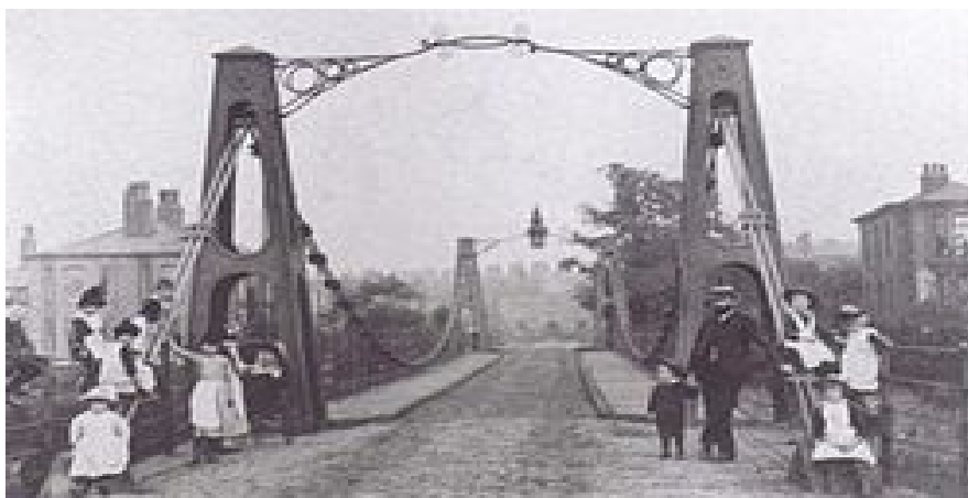
Figure 32. The Rebuilt Broughton Suspension Bridge.
