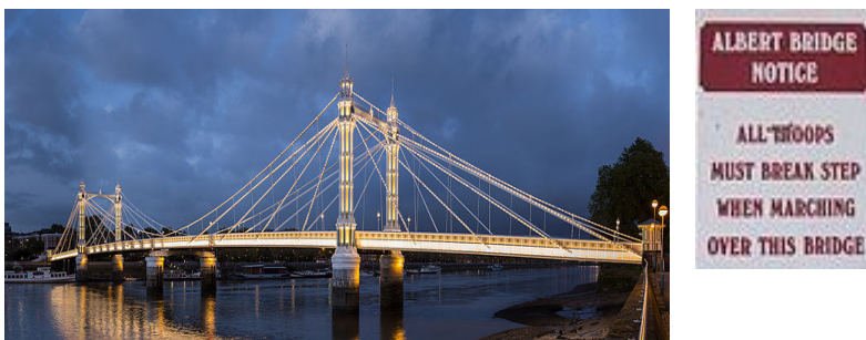
Figure 33. The London Albert Bridge.
