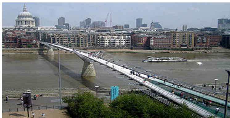
Figure 36. The London Millennium Foot-Bridge.
